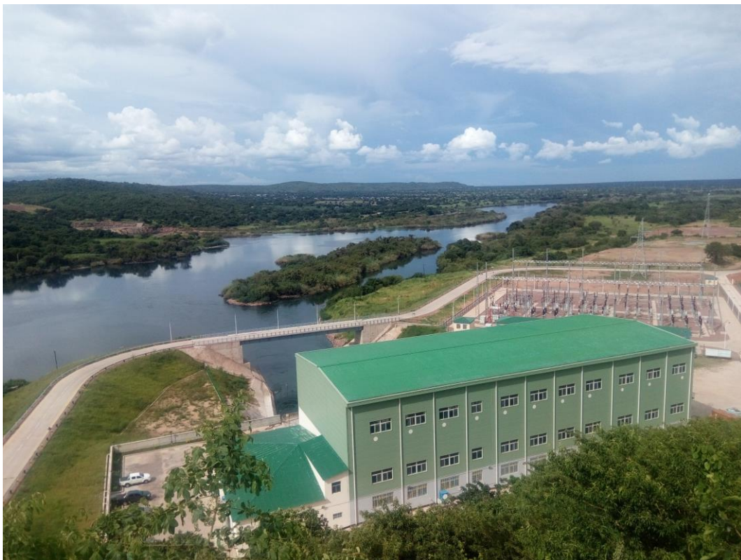
Figure 2: View of the completed hydropower station
